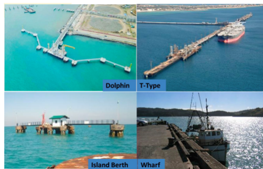
Figure 1. Types of Jetty Fuel Port Profile
